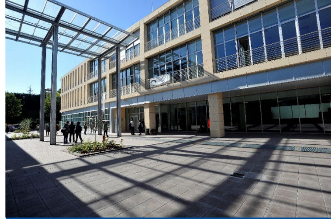
ENGINEERING AND IT DEPARTMENT UNITN UNIVERSITA' DI TRENTO Povo, TN
