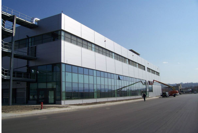
LOGISTIC BUILDING FERRERO SPA Alba, CN
