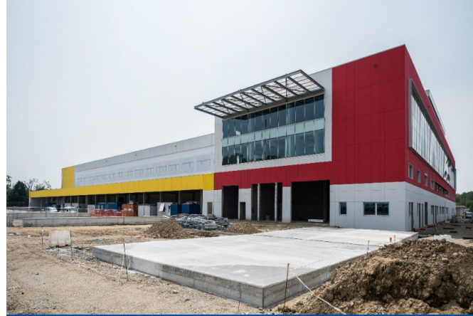
NEW BUILDING FOR DHL IN THE CARGO CITY AREA – MALPENSA AIRPORT DHL EXPRESS ITALY SRL Rozzano, MI
