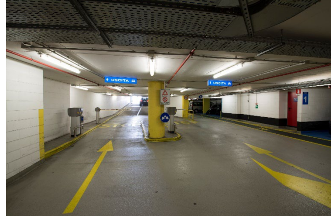
UNDERGROUND CAR PARK IN MEDA SQUARE PARCHEGGIO PIAZZA MEDA SRL Milan
