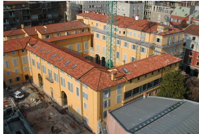
MILAN UNIVERSITY RENOVATION UNIVERSITA' DI MILANO Milan
