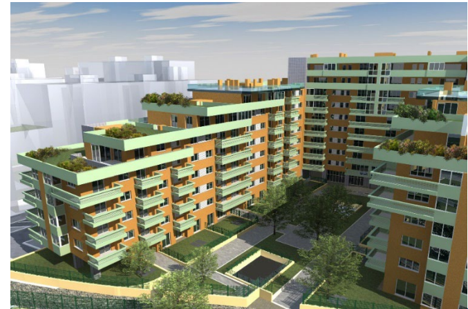
RESIDENTIAL COMPLEX IN VEROLENGO STREET CINQUE CERCHI SPA Turin
