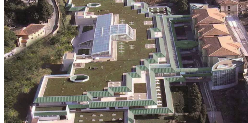
Client: Mayer Hospital Company Description: Construction New Children Hospital A. Mayer in Villa Ognissanti - Careggi - Florence
