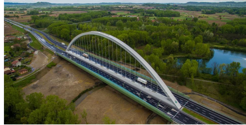
Client: A.T.I.V.A. S.p.A. Description: Rehabilitation of the Marchetti Viaduct - A4/A5 Santhià-Ivrea
