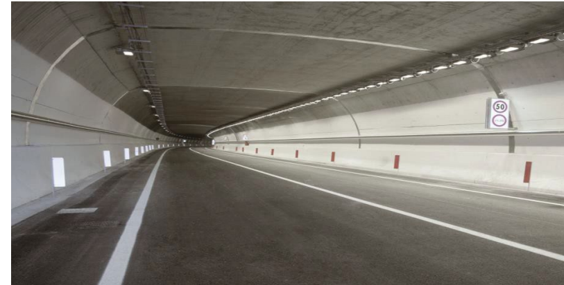
Client: Turin Agency 2006 Description: Construction of the Avigliana tunnel (tunnel 1.750 ml) - Avigliana (Turin)
