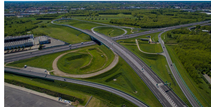
Client: Pedemontana Lombarda S.p.A. Description: Construction of the Highway Pedemontana Lombarda
