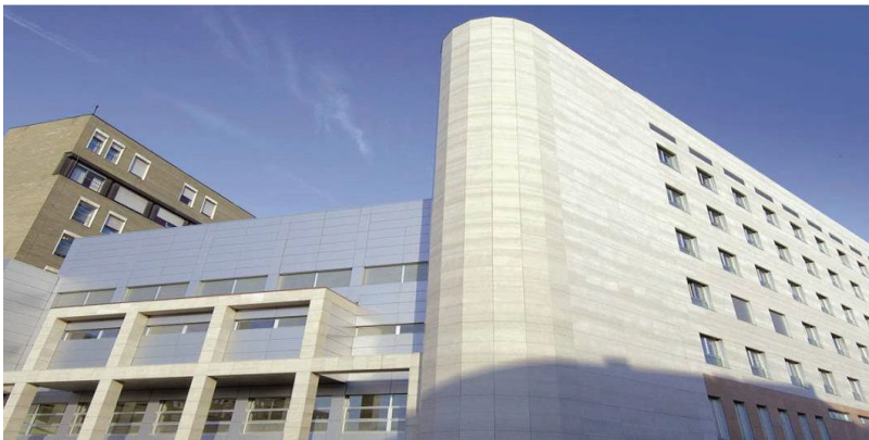
Client: San Donato Group Description: Enlargement Policlinic Hospital - S. Donato M.Se (Milan)
