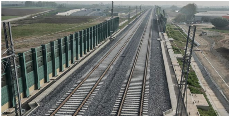
Client: CEPAV DUE Description: Construction of the railway connection HS/HC, stretch Treviglio-Brescia
