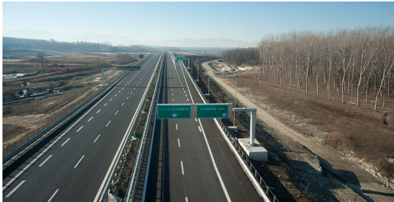
Client: ANAS S.p.A. Description: Construction of the Highway A33 Asti-Cuneo Lot 1.1
