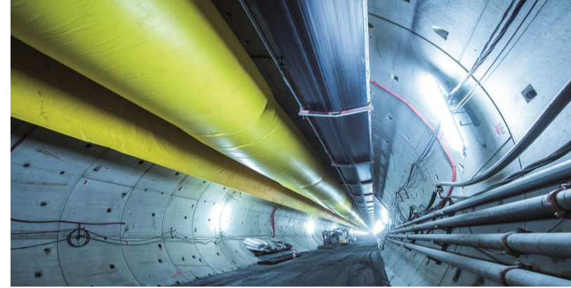
Client: S.I.T.A.F. S.p.A. Description: Construction Frejus safety tunnel - Bardonecchia (Turin)
