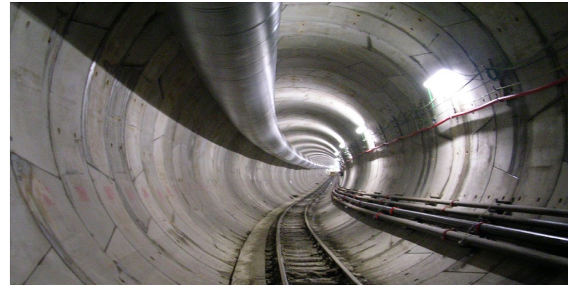
Client: M.N. Metropolitana di Napoli S.p.A. Description: Construction works Dante- Garibaldi route, Secondigliano warehouse and workshop, Piazza Dante station and Montesano corridor- Line 1
