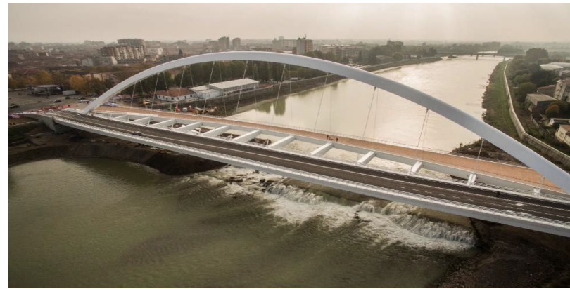
Client: Alessandria Municipality Description: Construction of the Meier Bridge
