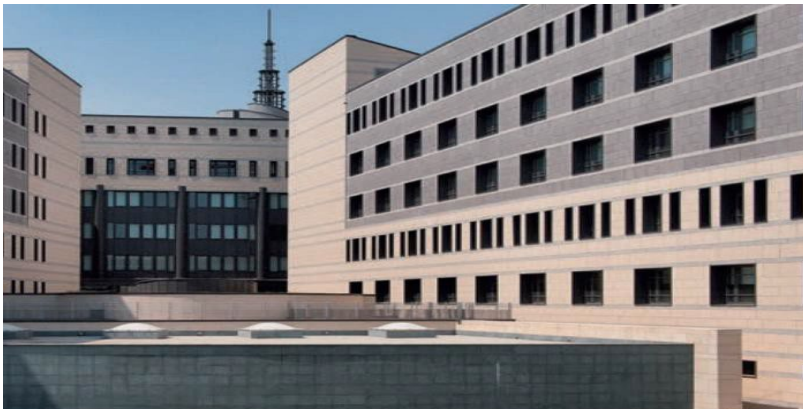
Client: Ministry of Justice Description: Construction of new Courthouse buildings - Vicenza
