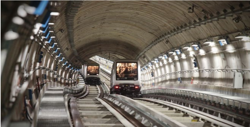
Client: Gruppo Torinese Trasporti S.p.A. Description: Construction of driverless metro in Turin Lots 3 and 5 - stretch Collegno-Porta Nuova (tunnel 5,300 m)
