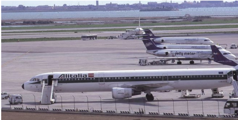
Client: SAVE S.p.A. Description: Rehabilitation runways, apron and hangar construction Marco Polo Airport - Venice - Tessera
