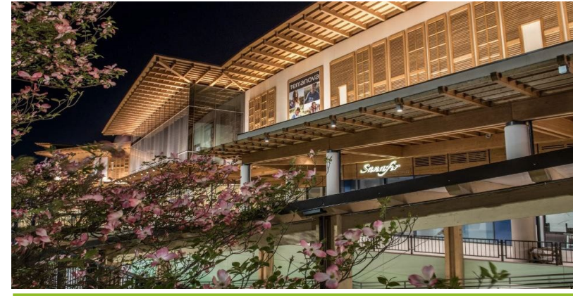
Client: T.E.A. S.p.A. Description: Construction Arese Mall - Arese (Milan)
