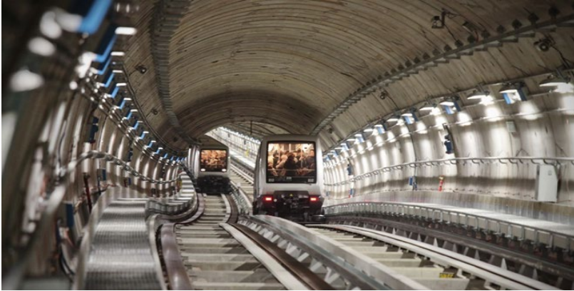
Client: Gruppo Torinese Trasporti S.p.A. Description: Construction of driverless metro in Turin Lots 3 and 5 - stretch Collegno-Porta Nuova (tunnel 5,300 m)
