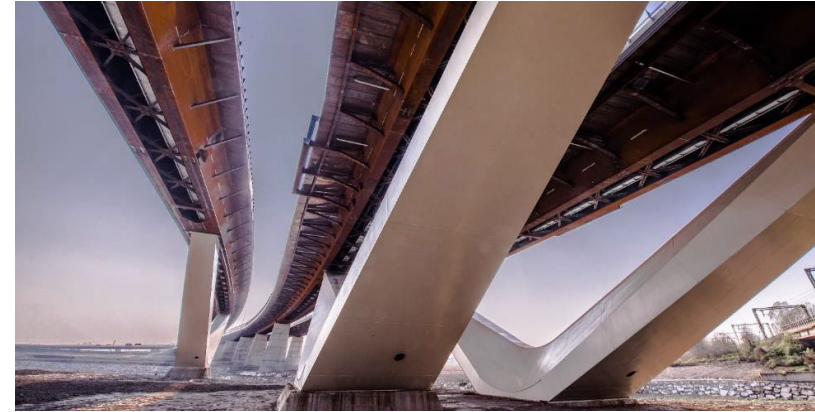
Client: C.A.L. Description: Construction of the External East Ring Road - Milan
