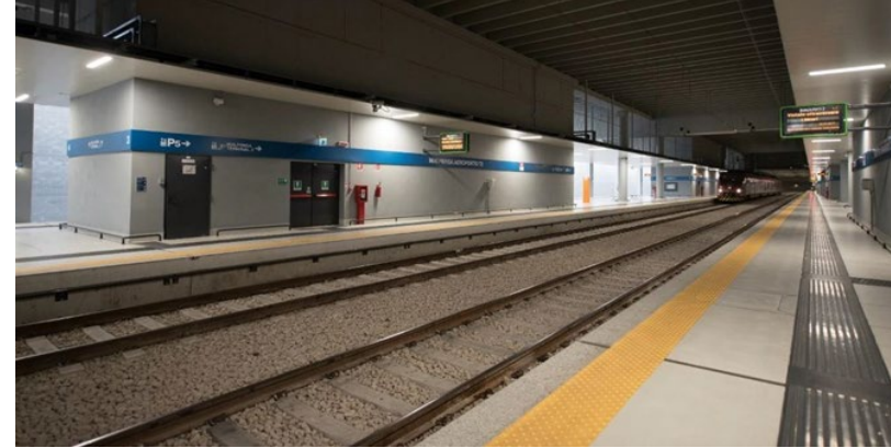
Client: Ferrovienord S.p.A. Description: Railway connection T1-T2 at Milano Malpensa Airport
