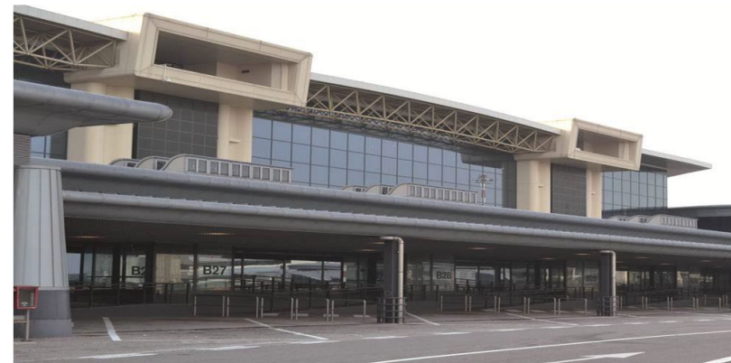
Client: S.E.A. S.p.A. Description: Construction Apron, service roads, terminal enlargement construction of ENAC Blg-Milano Malpensa Airport -Terminal 1
