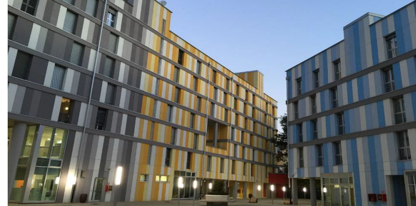
Client: Erasmus Fund Description: Construction of University Accommodation - Turin
