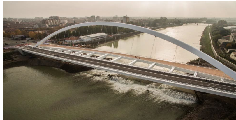
Client: Alessandria Municipality Description: Construction of the Meier Bridge
